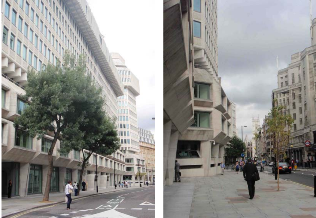
Petty France, SW1: The proximity of trees to buildings needs to be considered. The pavement space available for these new plantings (right) is more suitable than that available for existing trees (left).
