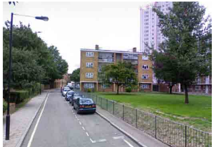
Crompton Street: open space plantings (sourced from Google Street View)
