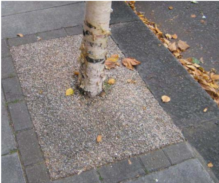
Pimlico, SW1: Neat, safe, maintainable simplicity is achieved by using resin-bound aggregate.
